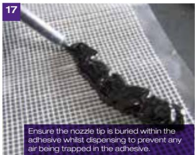
Apply the adhesive to the reinforcing mesh with the plastic backing sheet in place as per the picture keeping the end of the nozzle buried in the adhesive.
